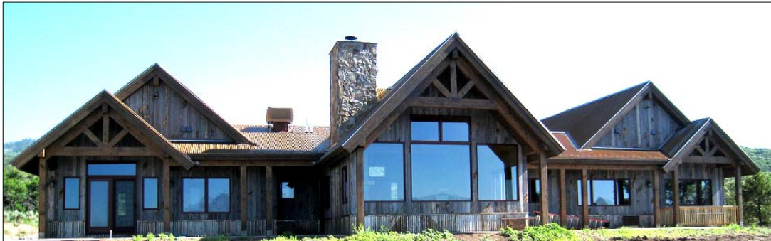
Exterior elevation of the custom home
