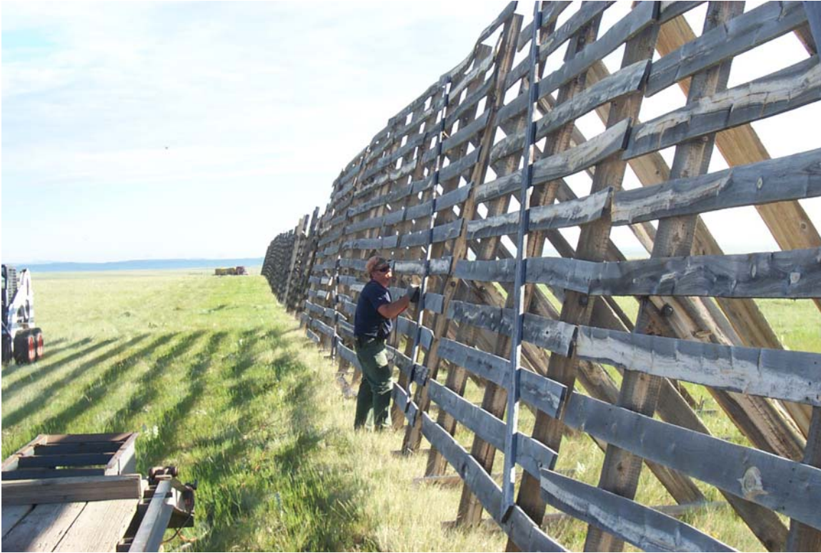
Centennial Woods crews dismantling snow fence near Laramie, Wyoming
